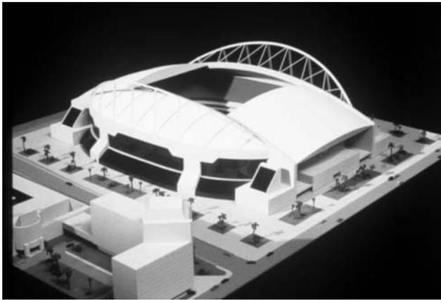
Fig.19. Retractable Roof for Phoenix Stadium Horst Berger's Design 1983
