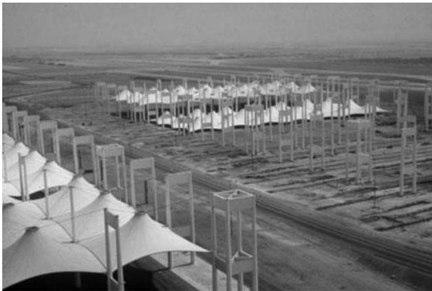
Fig.10: Jeddah Construction: Module A to E up in place, Module F up, G being installed
