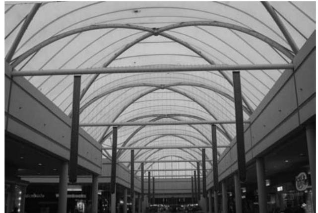
Fig.17. Silicone Coated Fiberglass Fabric at Poughkeepsie Mall. Horst Berger Part. Eng.
